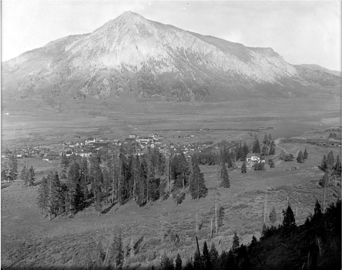
Figure 4 Crested Butte, Colorado in early 1900's with Coal Creek in foreground. "Courtesy, History Colorado (Denver & Rio Grande Collections, Scan # 20004344)"
